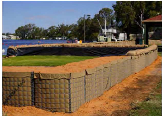
The DefenCell flood levee near the Renmark Club on Murray Avenue, (ABC News - Evelyn Manfield). Reproduced by permission of the Australian Broadcasting Corporation © 2023 ABC
