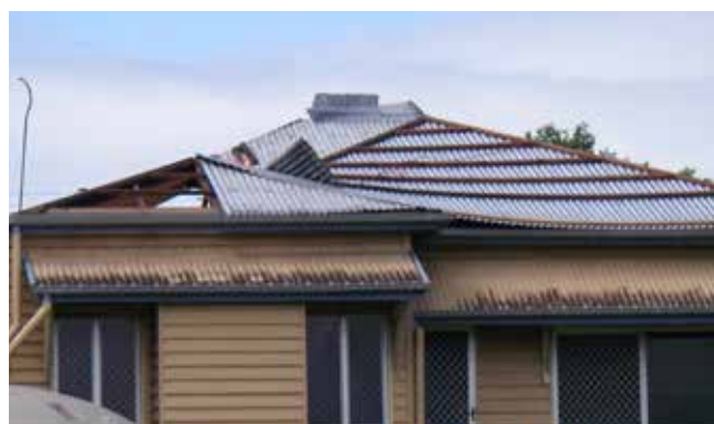
Figure 2: Removal of roof cladding and battens from windward face.
