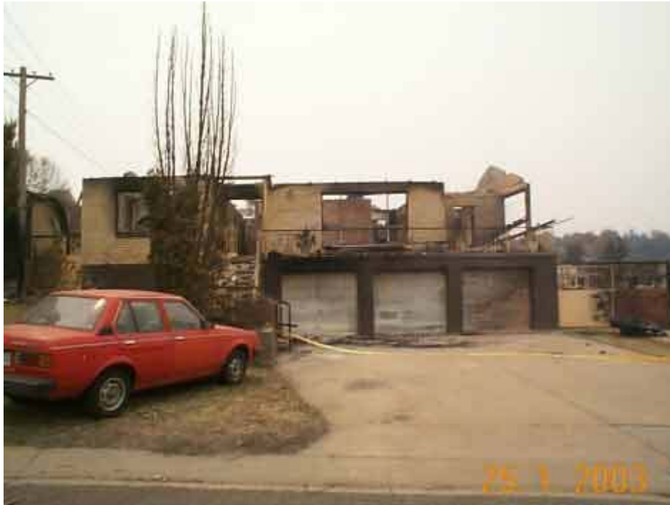
A two storey house in Duffy completely destroyed.
