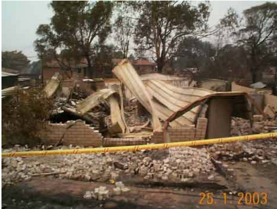
Gutted house in Duffy.
