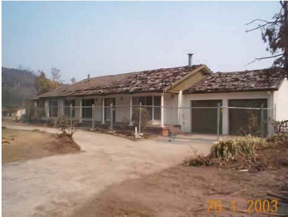
This home in Chapman was extensively damaged by the high winds.
