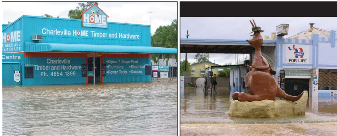
Figure 5.2. Business premises flooded in Charleville (Photo source: Charleville Home Hardware and Chester Wilson)
