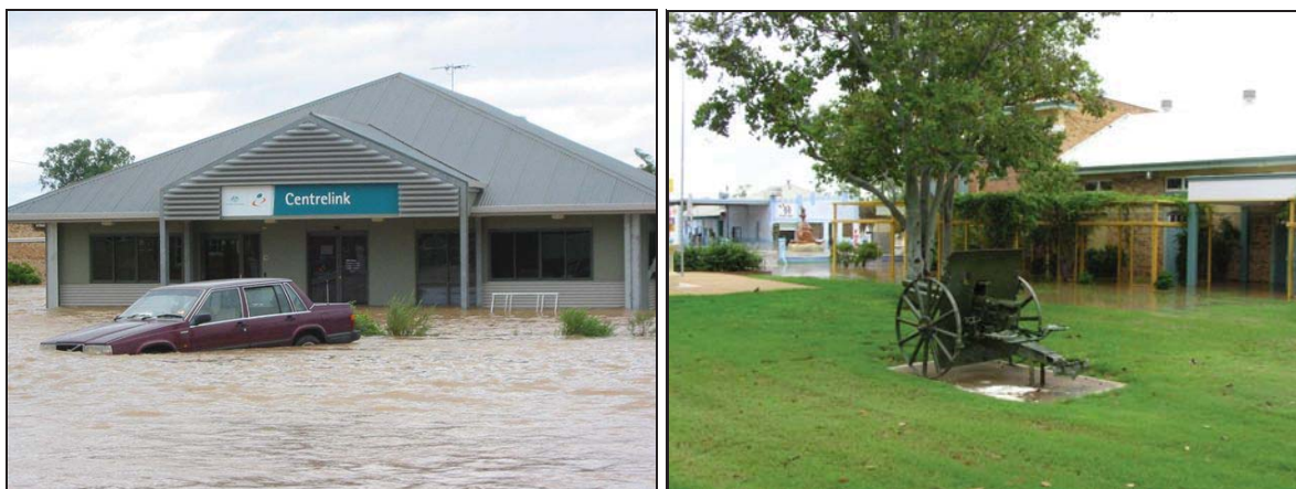
Figure 5.3. Buildings of institutions flooded in Charleville (Photo source: Carol Finlay and Chester Wilson)
