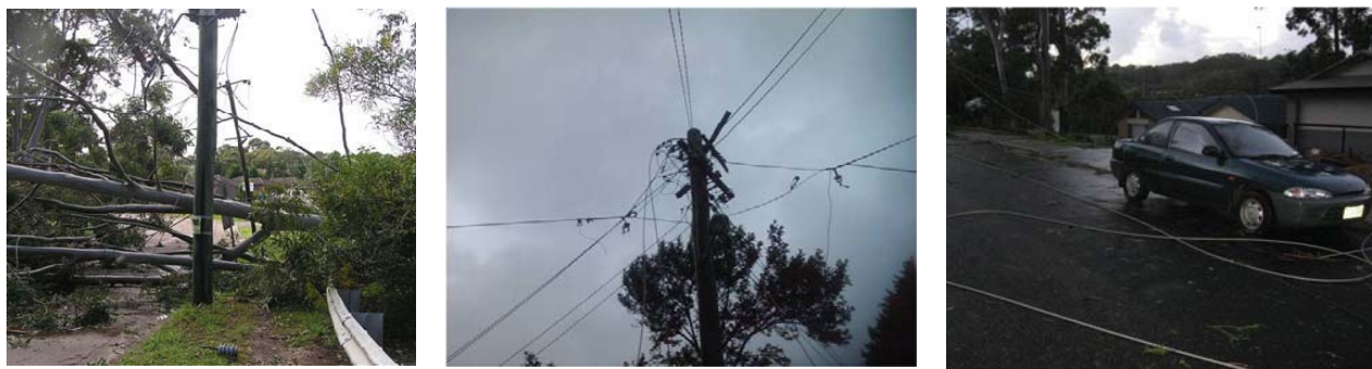
Figure 12 Damage caused to power lines during the storm. Source: Images courtesy of Energy Australia).
