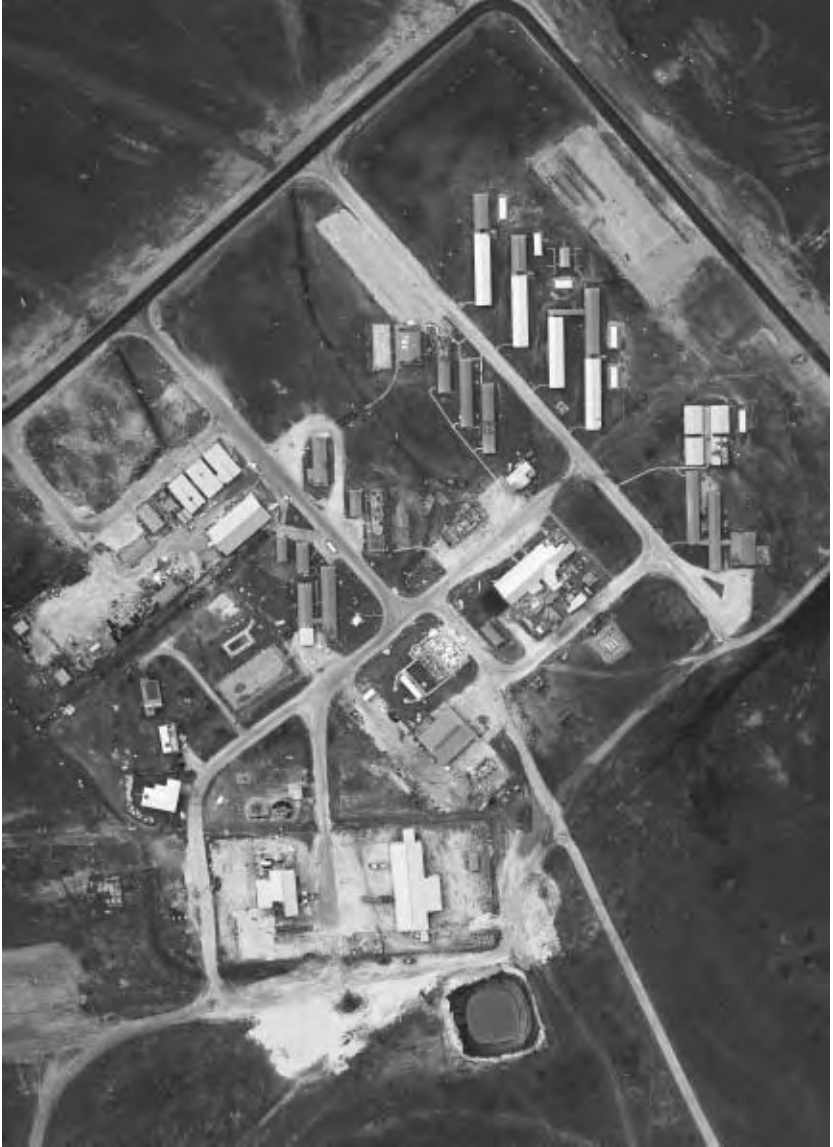
Figure 6-3: Vertical Photograph—Cyclone Damage RAAF Base Learmonth, Western Australia, October 1999. (RAAF Photograph)
