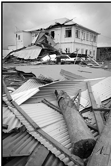
Figure 3:1 Debris caused by Tropical Cyclone Larry – March 2006
