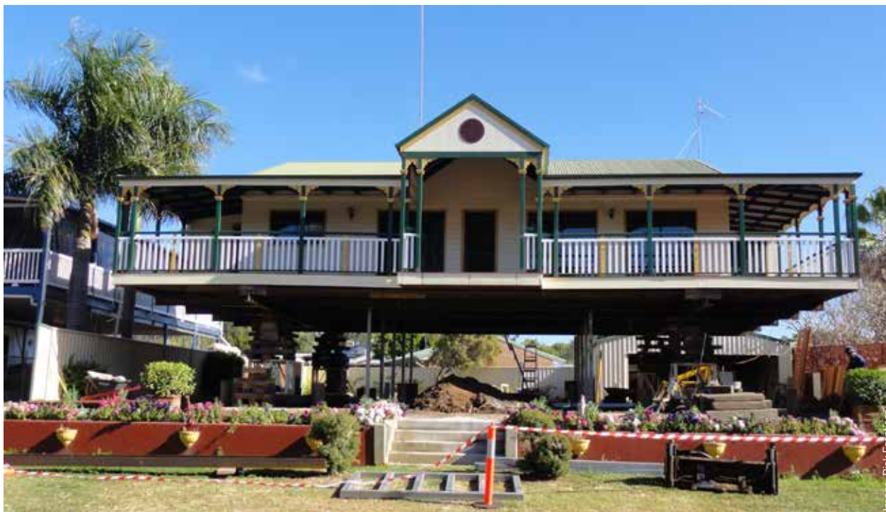
The process of raising houses in flood-prone areas is complex and expensive.
