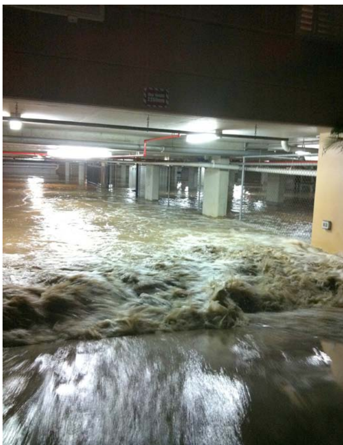
Floodwaters inundate car park of Regatta Apartments (photo courtesy Paul Rees)
