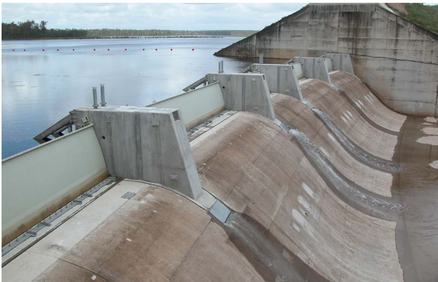
Crest gates on the spillway of Lenthalls Dam (photo courtesy Wide Bay Water)
