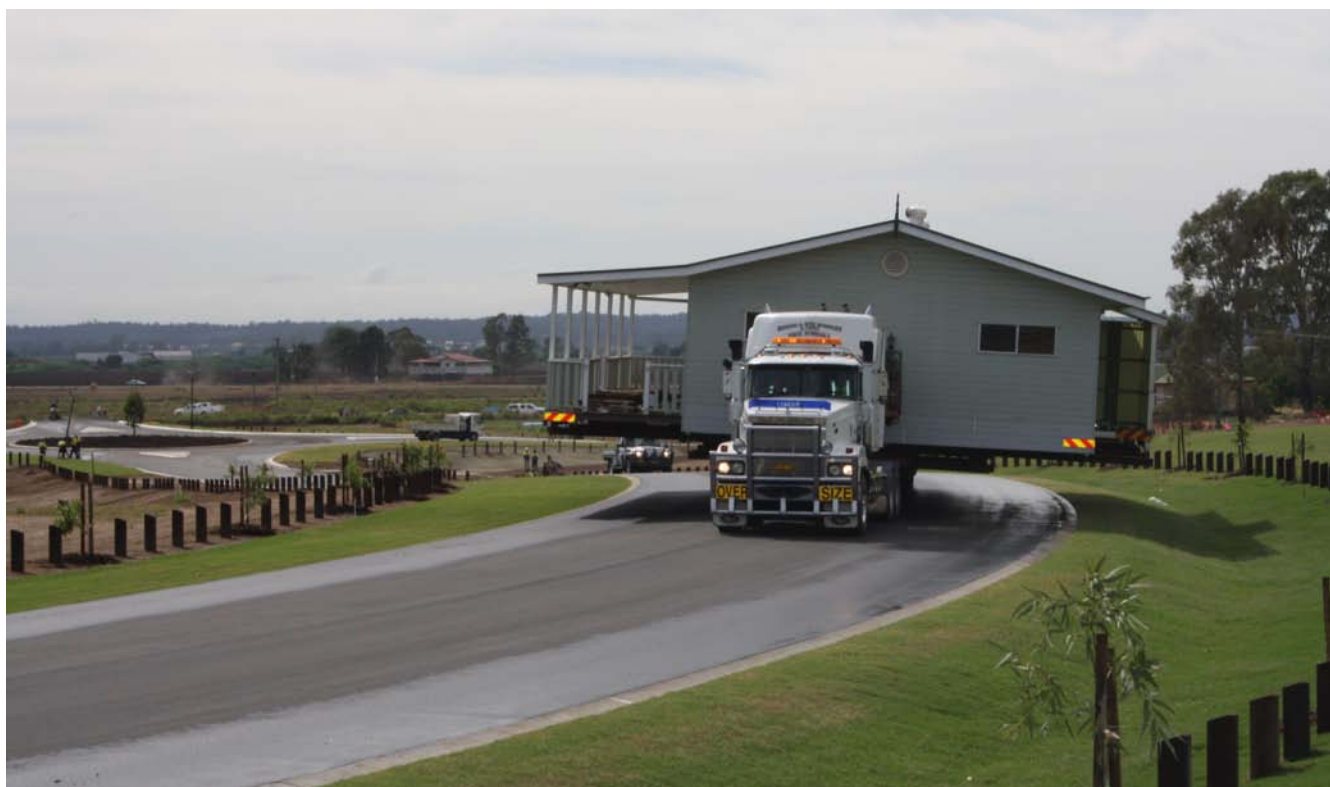
Grantham house being relocated to higher ground (photo courtesy Lockyer Valley Regional Council)
