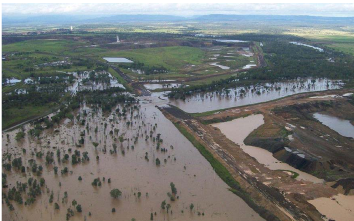
Rolleston Coal Mine, 2010/2011 floods (photo supplied)
