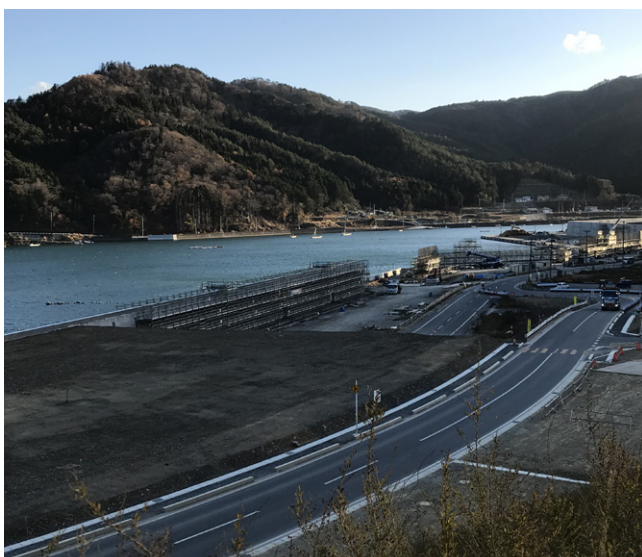
The government has built sea walls to protect coastal communities. The tsunami reached 21 metres high in this area.
