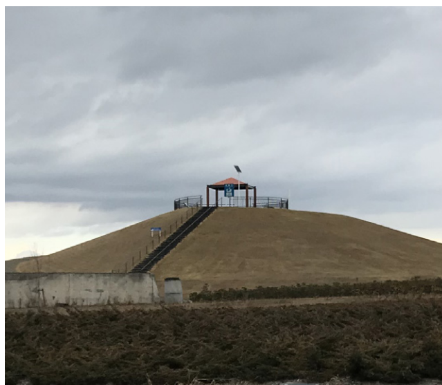
A 'Hills of Hope' near Sendai airport. The path at the left provides better access for disabled people. The hill is 11 metres high and exceeds the height of the tsunami recorded in this area.
