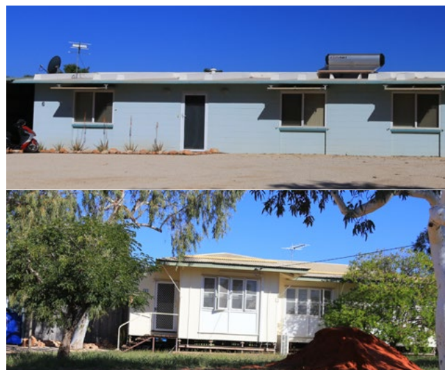
Typical U.S. Navy block house (above) and 1960s-era fibro house (below) in Exmouth.
