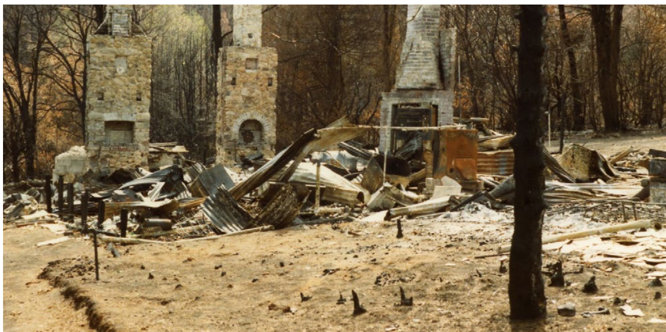
Remains of a house in Mount Macedon, Victoria after the Ash Wednesday bushfires in 1983 when 180 fires caused widespread destruction across Victoria and South Australia.
