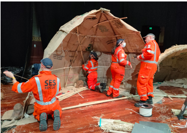
Refuge 2021: Displacement. SES personnel building a temporary shelter.
