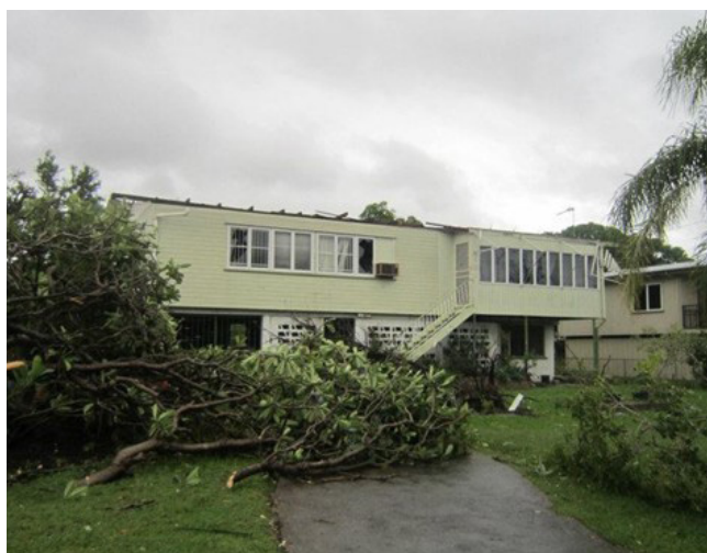
Destruction caused by a tornado in Townsville, Queensland, 20 March 2012.
